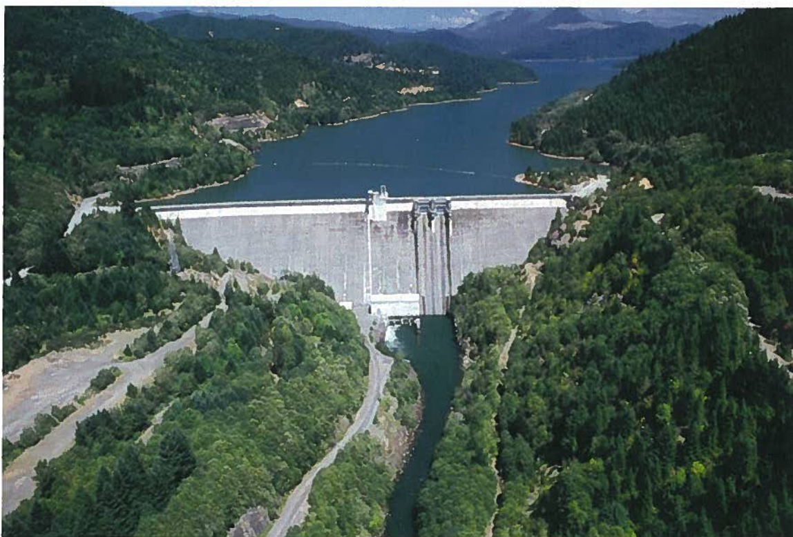
Green Peter Dam and Reservoir
